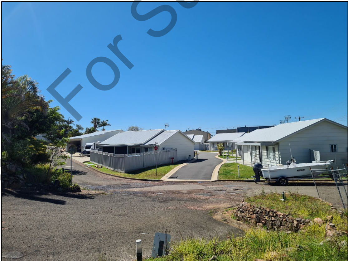
Below: Current entry roads looking east towards upgraded roads and renovated cabins.
