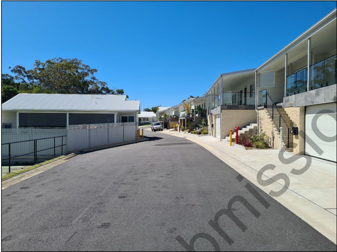
Above: Southern road (Angel Close) looking east
